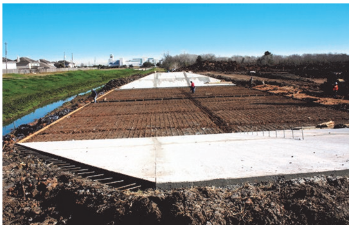
A weir is being built on Mud Gully channel in the South Belt area.
