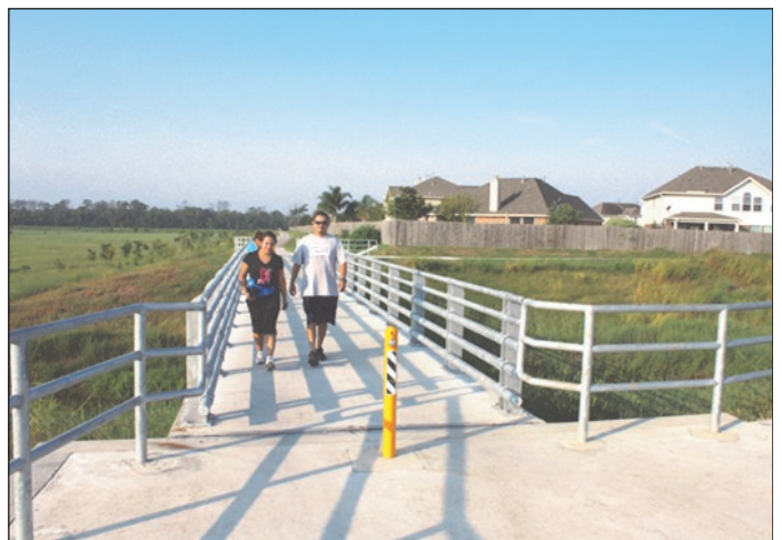
Walkers use the recently completed 8-by-130-foot pedestrian bridge that spans a drainage ditch in the Dixie Farm Road Park.
